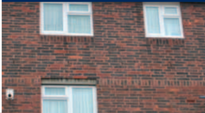
Windows at Andover - AFTER
