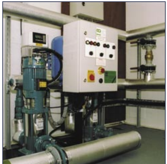
New equipment like this water booster may need to be installed in some locations.
