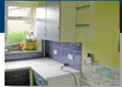
Work in progress on a new kitchen
