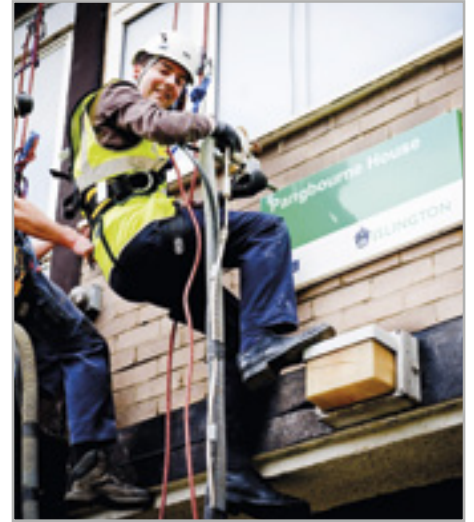
Councillor Murray helps to install cavity wall insulation
